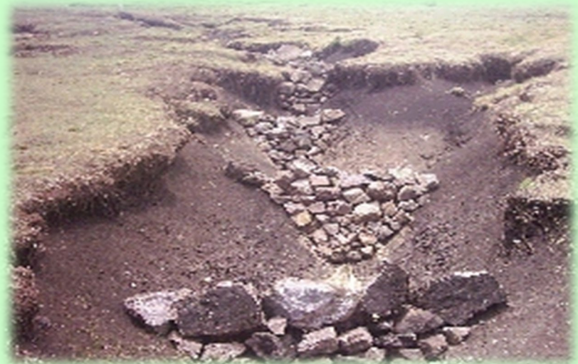
CONTROL DE CARCAVAS
